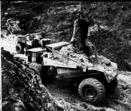
Draglines of 4 and 5 cubic yard capacities load Tournapulls with wet bauxite ore. These pits, about 18.6 miles south of Paramaribo, Surinam, are owned by Billiton Bauxite Mines, of Surinam's Billiton Company.
